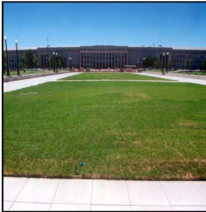
Photo 2-23. Green Roof at the Pentagon Remote Delivery Facility
