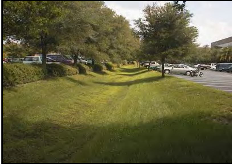
Photo 5-7. Vegetated Swale Adjacent to Impervious Parking Lot
