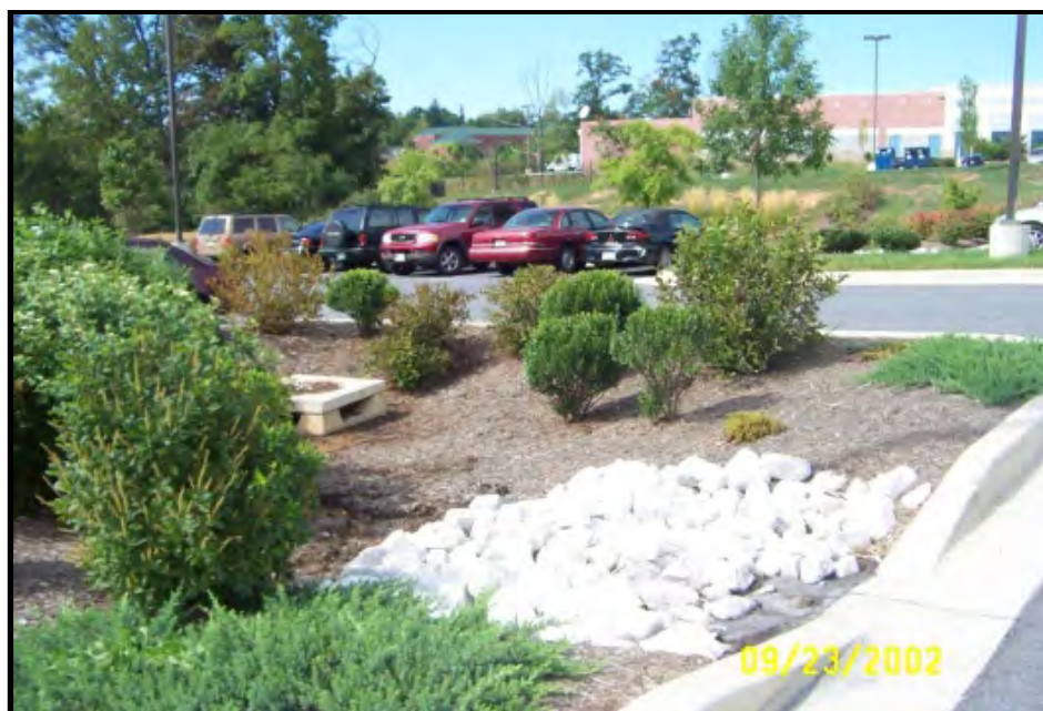
Photo 5-3. Inflow Entrance - Curb Cut with Riprap
