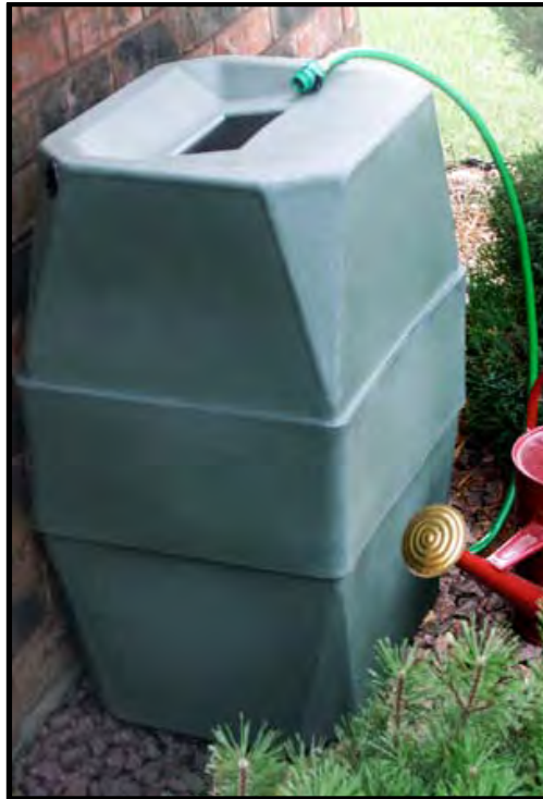
Photo 5-19. Residential Rain Barrel
