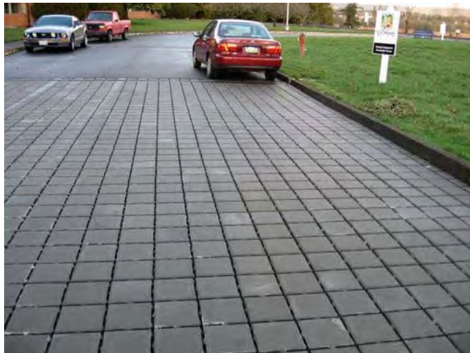
Photo 1-8: Permeable Pavement
