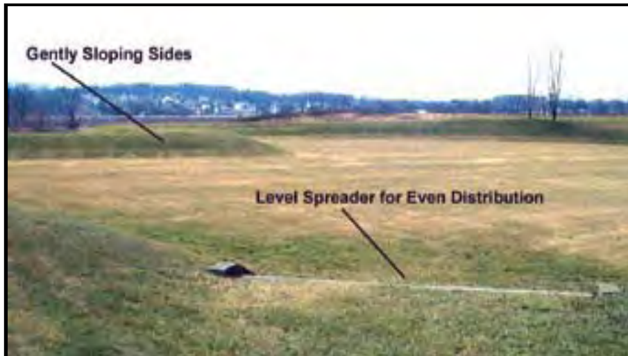
Photo 2-25. Infiltration Basin (Source: SEMCOG, 2008)
