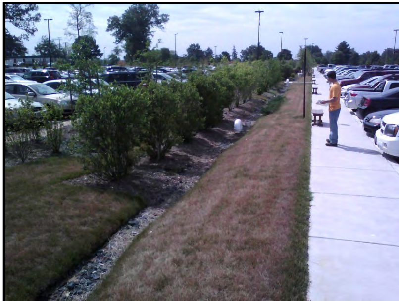
Photo 5-10. Typical Bio-Swale
