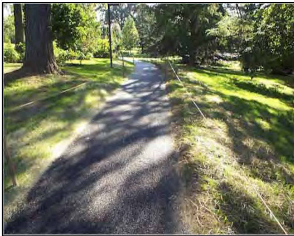
Photo 5-17. Porous Asphalt Along Pedestrian Walkways
