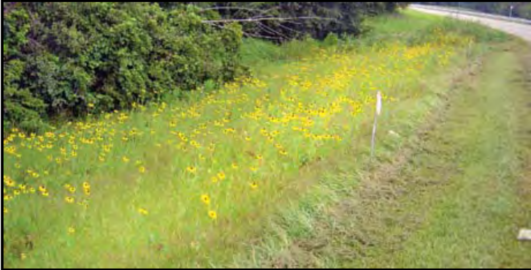
Photo 2-15. Vegetated Filter Strip Along Roadway (Source: SEMCOG, 2008)
