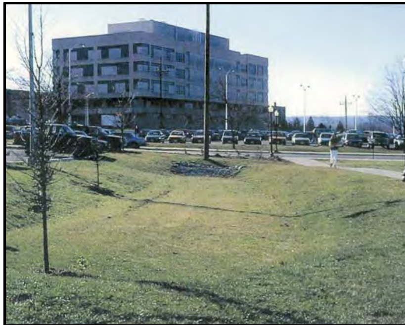
Photo 5-8. Vegetated Swale in a Commercial Setting
