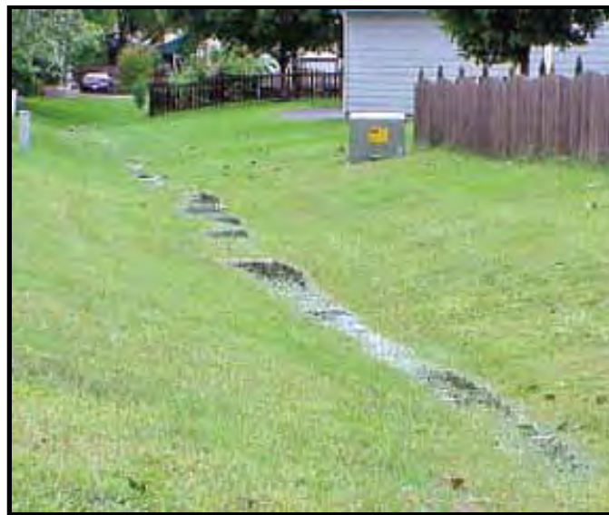
Photo 2-14. Grass Swale (Source: PA Stormwater IMP Manual, 2006)
