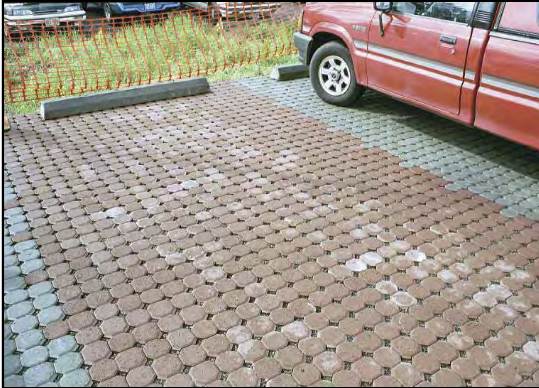
Photo 5-14. Permeable Pavers at Multnomah Art Center
